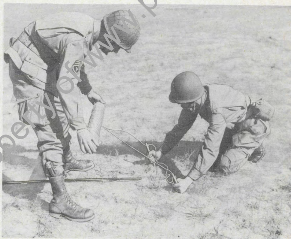
Step 7. Drive guy-wire stakes in ground near small end of mast.
