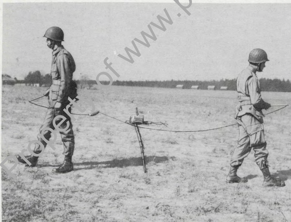
Step 9. Go five paces out from small end of mast, turn 90 degrees to the right, and go four paces. Drive the guy-wire stakes in securely, both men working at the same time.
