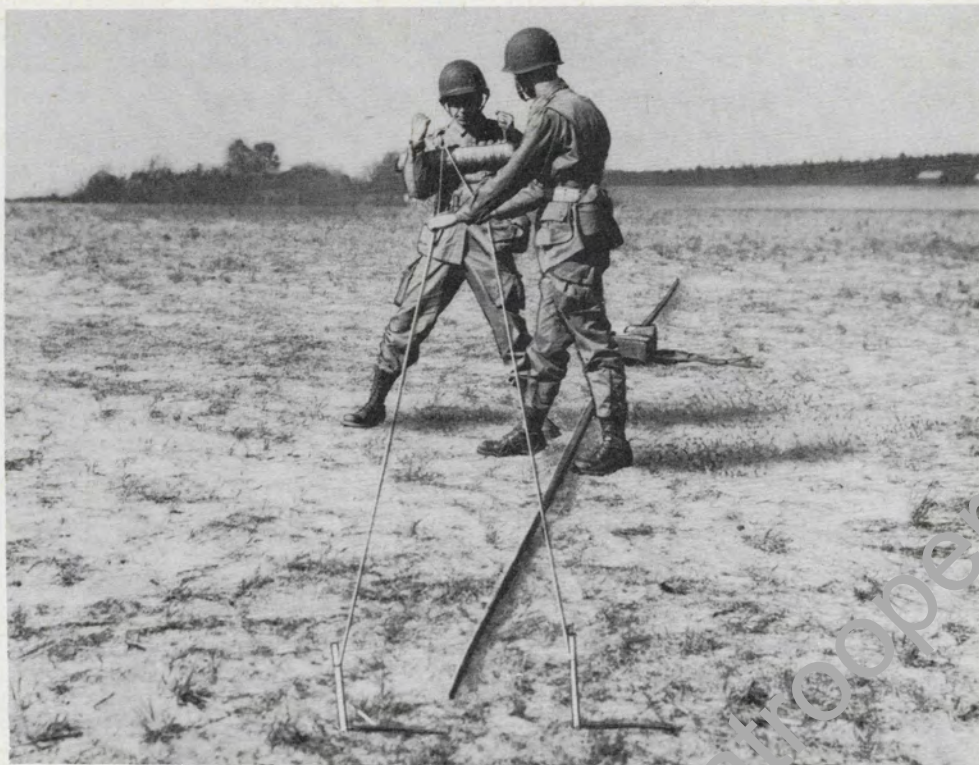
Step 8. Unroll guy wires. One man should unroll the wire and the other should keep the wires straight.
