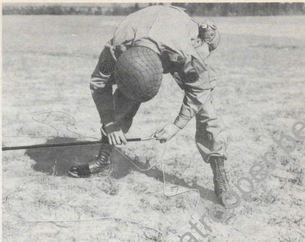
Step 10. Insert guy-wire assembly into top of antenna mast.
