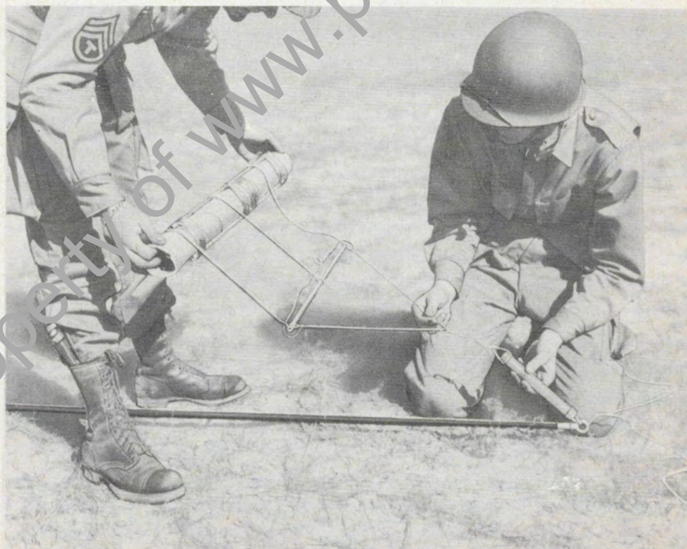
Step 11. Connect hook at end of flat top to guy-wire assembly.
