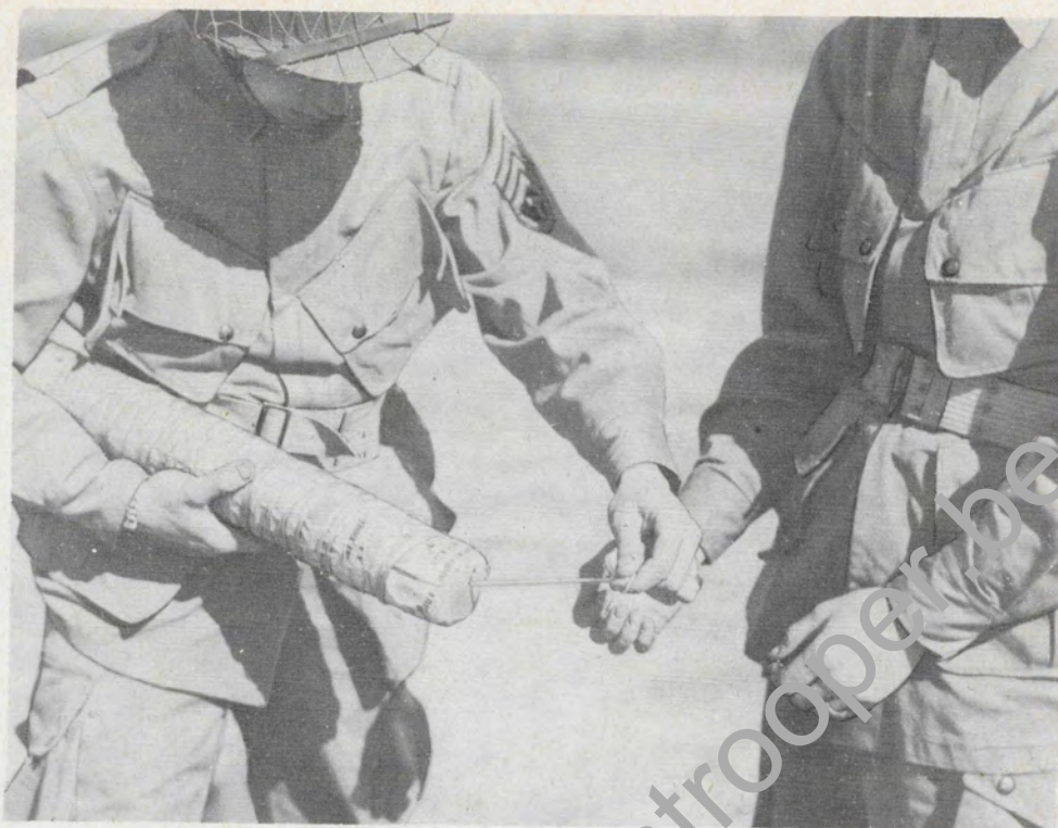
Step 6. Pull cord to open guy-wire antenna flat top assembly.
