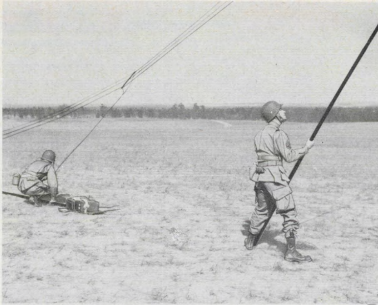
Step 12. Raise one mast. One man should hold other mast to prevent slipping or fouling of wires.
