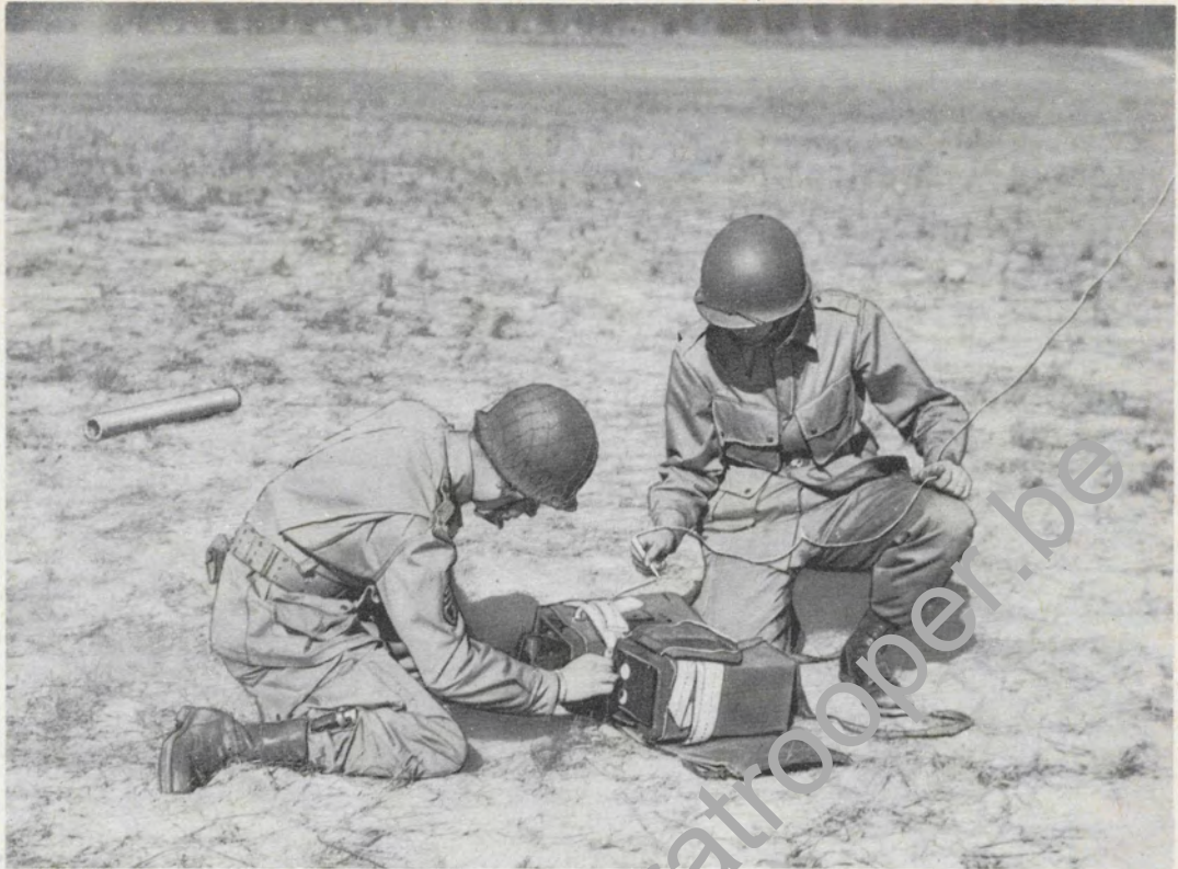
Step 14. Pull out counterpoise ribbons and insert antenna plug in antenna jack.
