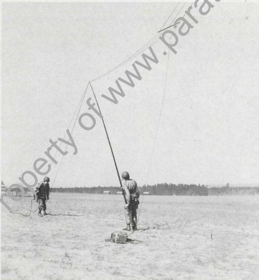
Step 13. Raise other mast carefully. Watch tension of antenna flat top and slack in guy wires.
