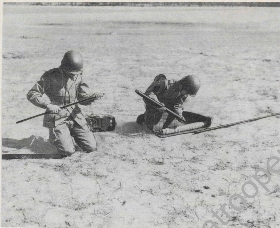
Step 4. Fit sections of antenna masts together.
